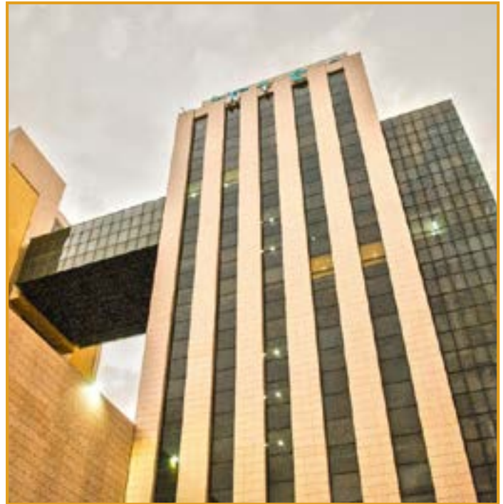
Empresarial Tower at Hotel Hesperia WTC Valencia. Photo credit: Hesperia WTC Valencia
